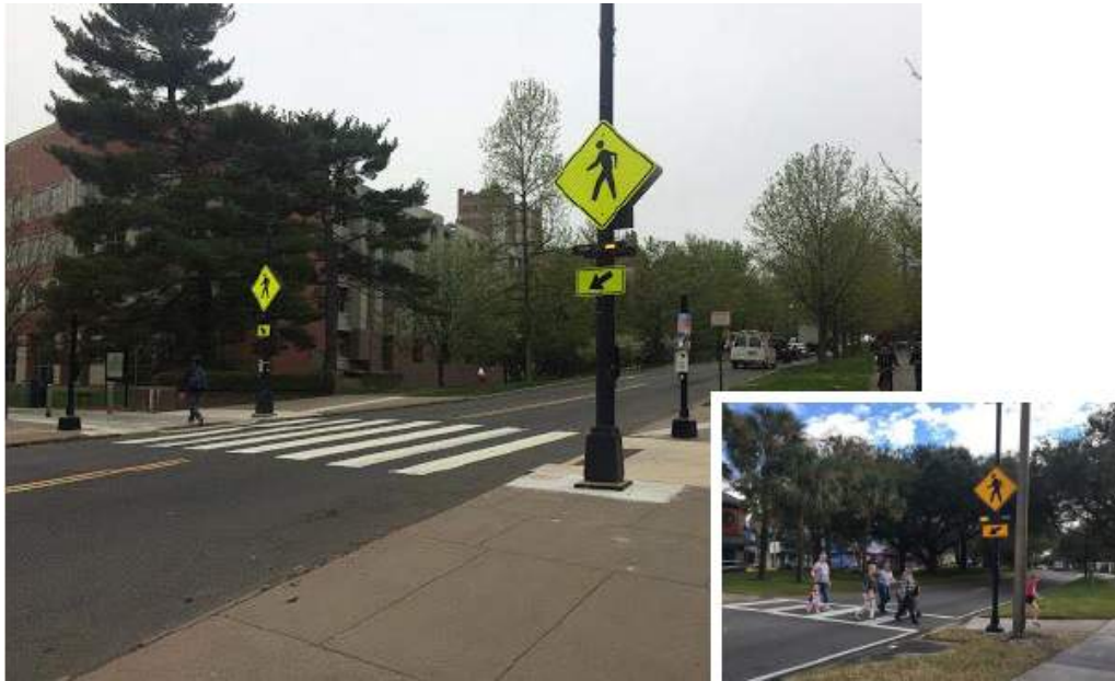
Rapid Rectangular Flashing Beacon (RRFB)
